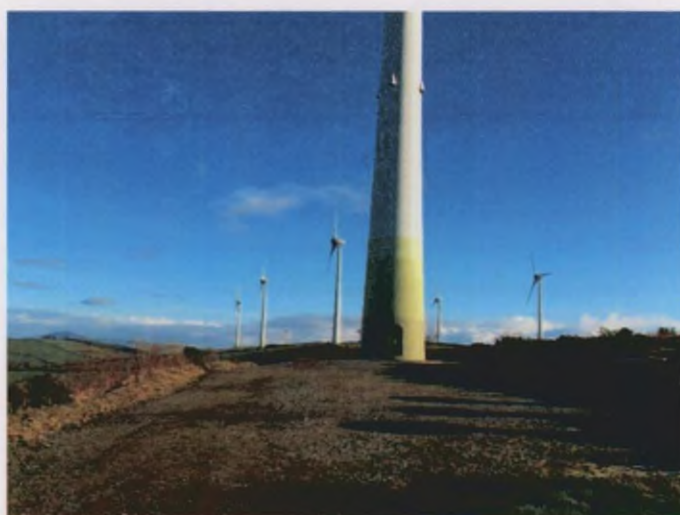
Plate 8: T8 and associated hardstand, looking ENE.
