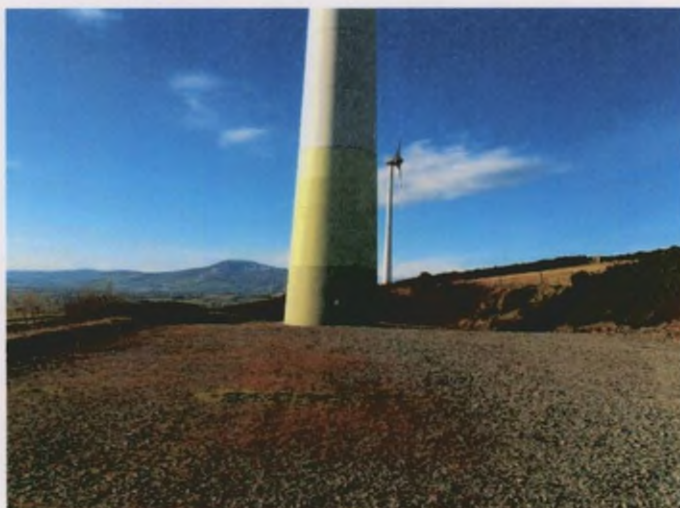
Plate 6: T6 and associated hardstand, looking W.
