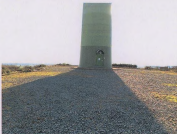
Plate 5: T5 and hardstand, looking S.
