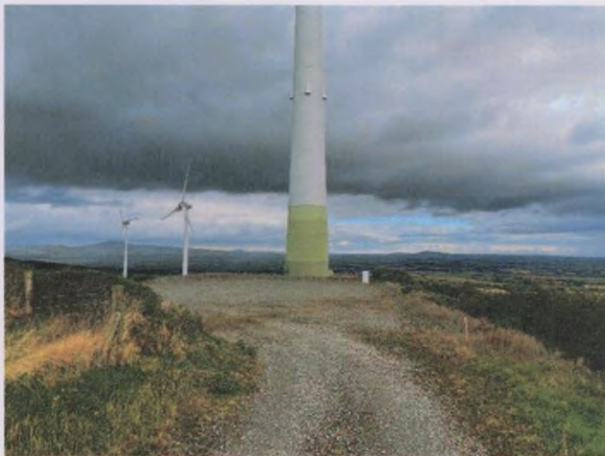
Plate 3: T3 and associated hardstand, looking NE.
