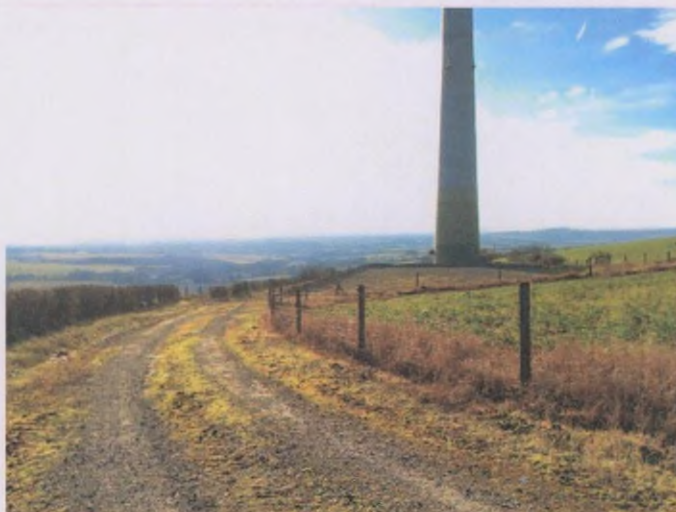
Plate 4: T4, hardstand and road to same, looking SW.
