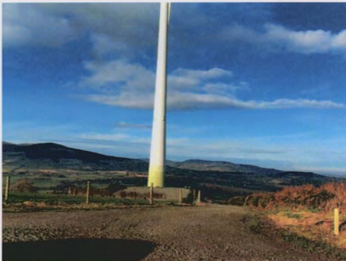
Plate 2: Existing T2 and road to same, looking NW.
