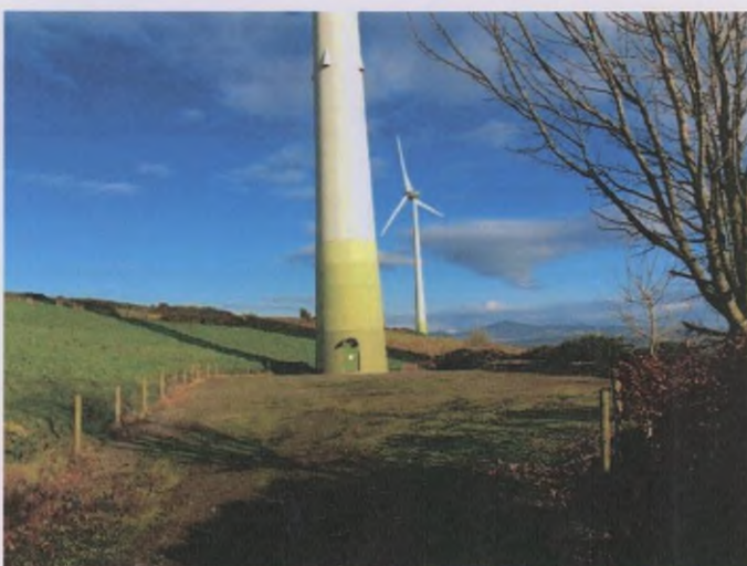
Plate 11: T11 and associated hardstand, looking NE.
