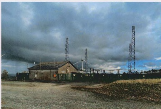
Plate 12: Existing substation, looking ESE.
