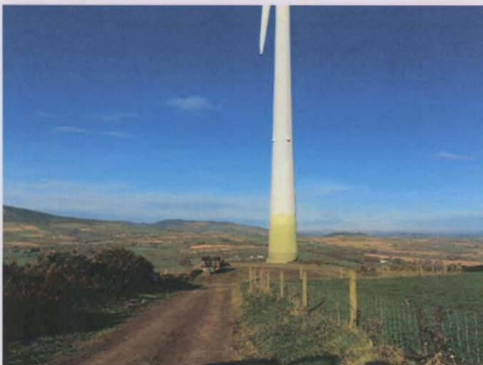
Plate 10: T10 and associated hardstand, looking NW.
