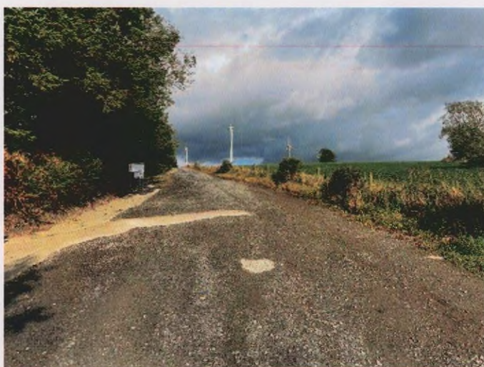
Plate 13: Existing entrance and road to wind farm, looking NE.
